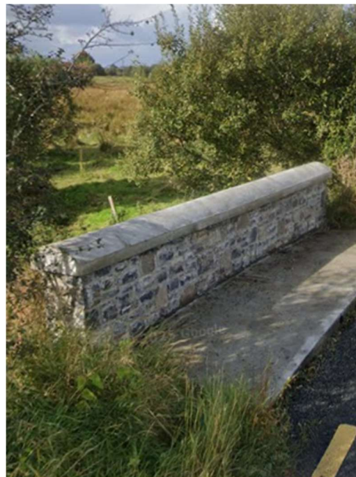
Figure 8: Bridge 1 - Wall View
