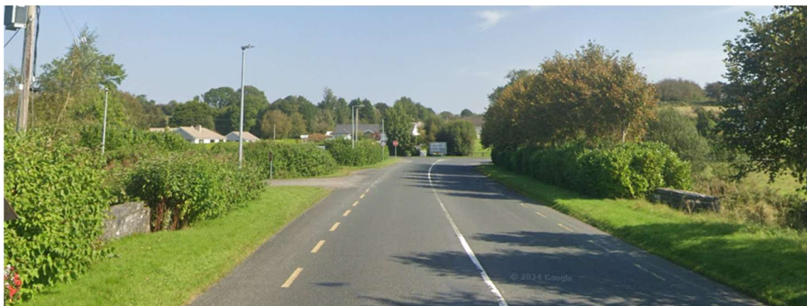
Figure 13: Bridge 3 - Google Street View ©2025 Google
