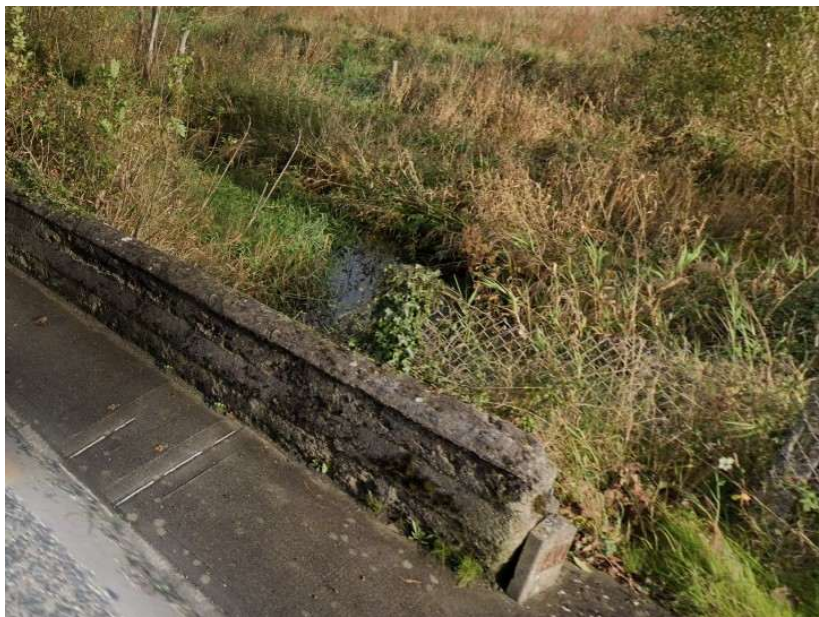
Figure 16: Bridge 6 - Google Streetview ©2025 Google
