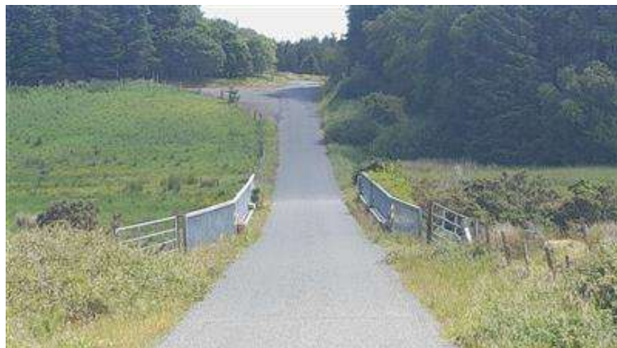
Figure 32: Bridge 15 - Road View
