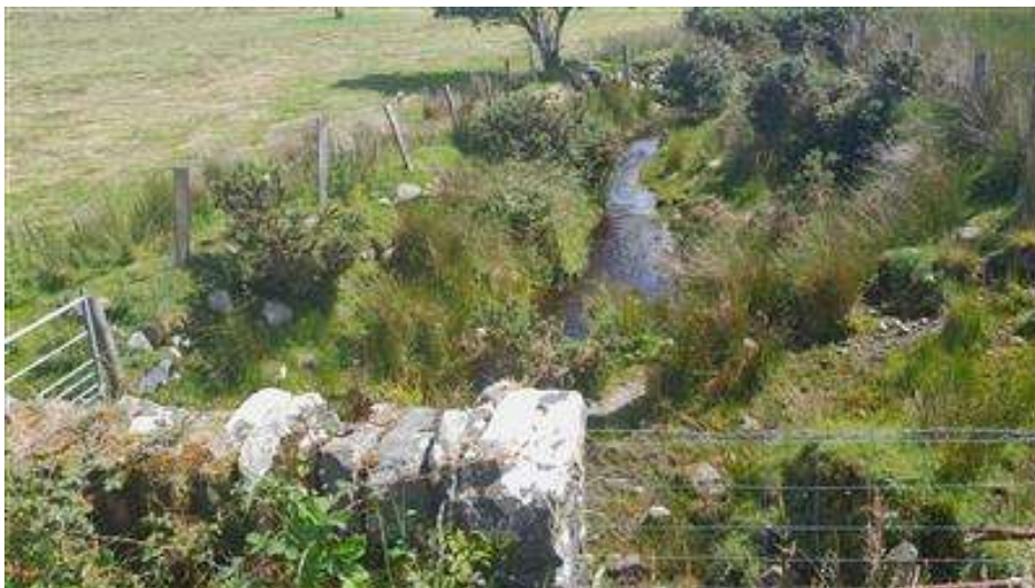
Figure 29: Bridge 14 - Wall View
