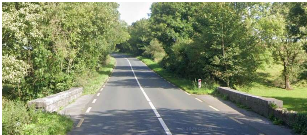
Figure 27: Bridge 12 - Google Maps Streetview ©2025 Google
