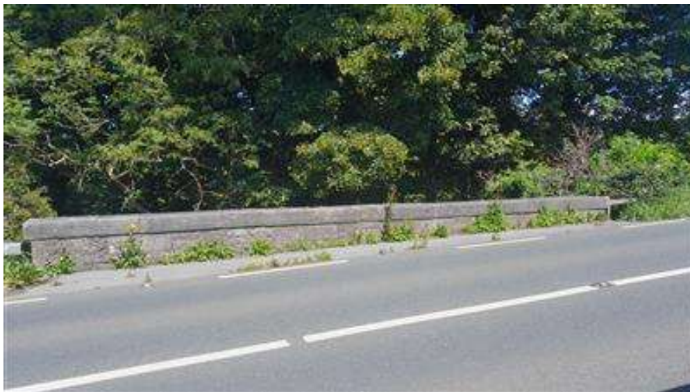
Figure 26: Bridge 12 - Roadside Wall View
