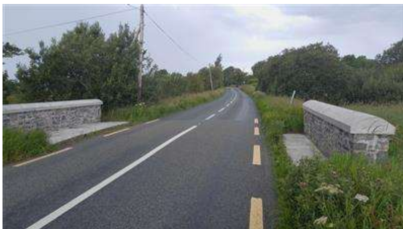
Figure 9: Bridge 1 - Road View
