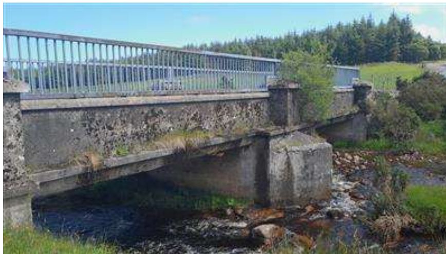
Figure 31: Bridge 15 - Elevation View
