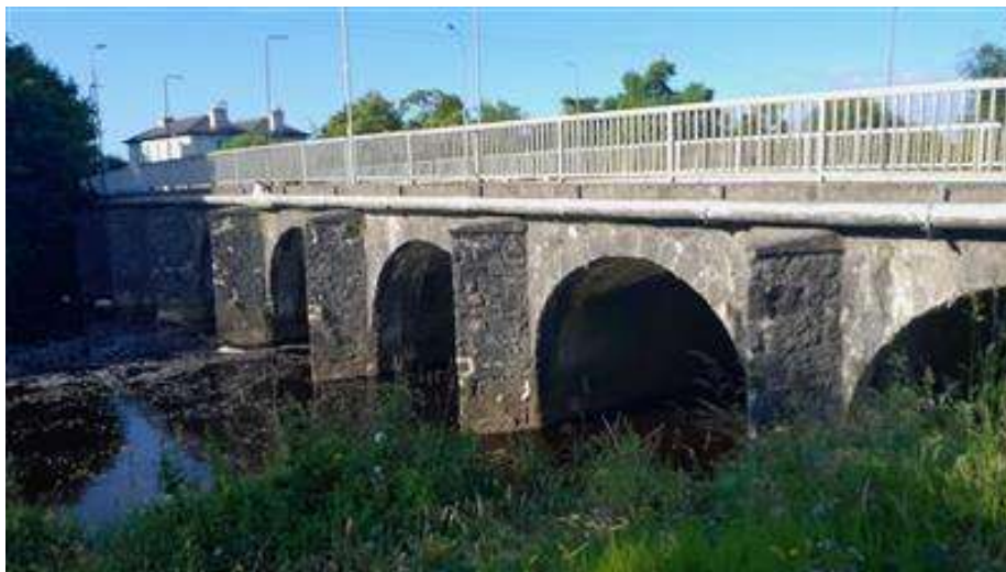
Figure 15: Bridge 5 - Elevation View
