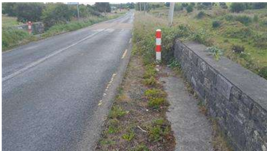
Figure 11: Bridge 2 - Wall View
