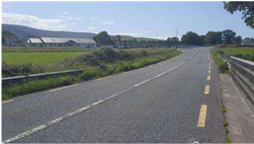
Figure 20: Bridge 9 - Road View
