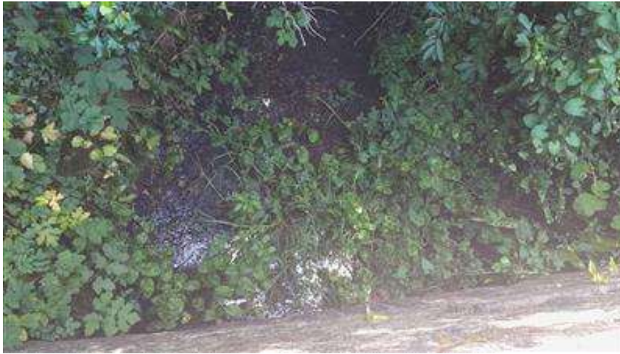
Figure 18: Bridge 8 - Over Bridge wall View
