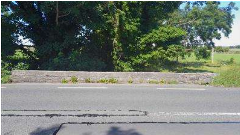
Figure 23: Bridge 10 - Bridge wall View
