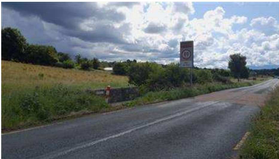
Figure 10: Bridge 2 - Road View
