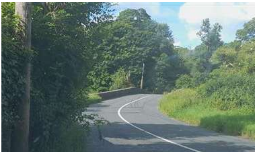
Figure 14: Bridge 4 - Approach from Road Bend
