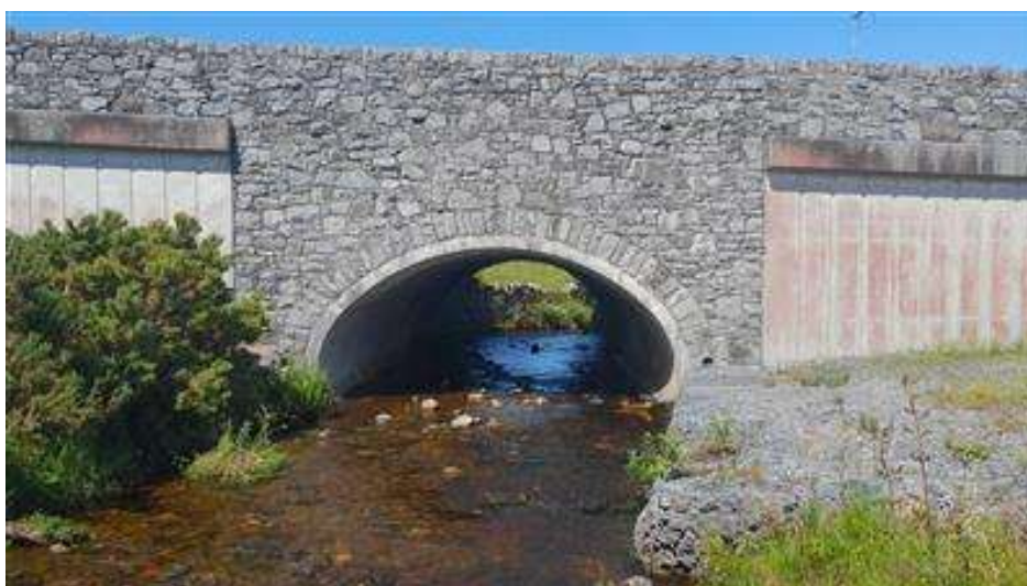
Figure 25: Bridge 11 - Elevation View
