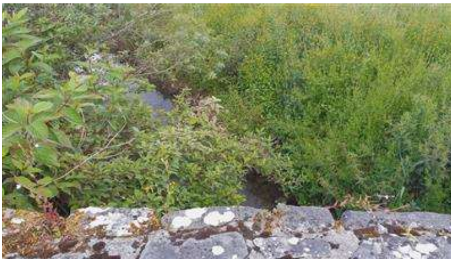
Figure 12: Bridge 3 - Over Wall View
