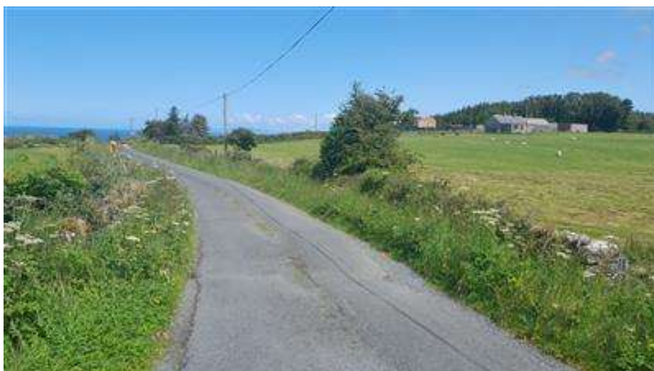
Figure 30: Bridge 14 - Road View
